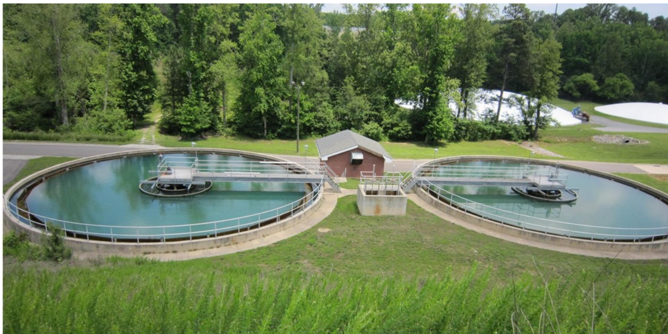
Water treatment site
